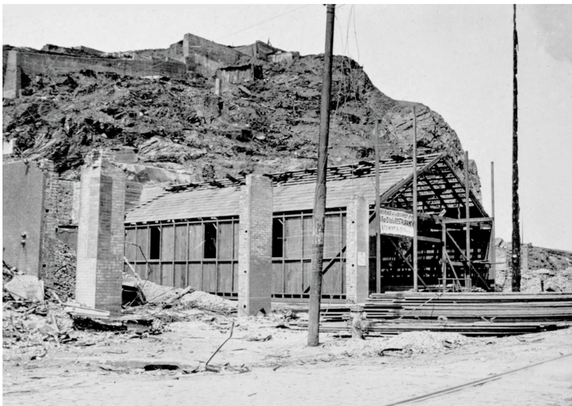
The temporary Fior d'Italia is in the midst of being erected
