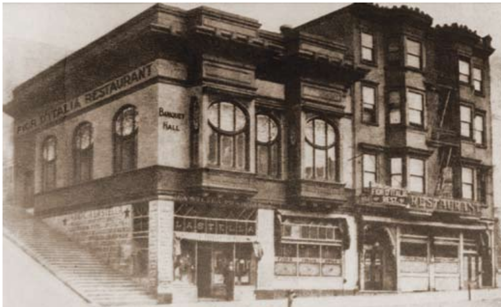
The Fior was rebuilt at 492 Broadway, the corner of Kearny, in 1909. Later, the restaurant Vanessi's took its place. The building still exists.
